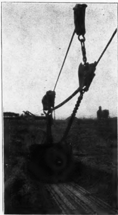
The Start of the Digging
